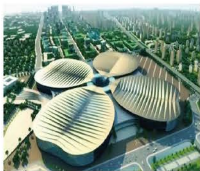
上海国展中心高空间照明采用ACDrV驱动的High Bay 灯具 Shanghai Nation Center Adopts High Bay lighting based on ACDrv
