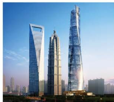
上海中心外立面照明采用ACDrV的投光灯 Shanghai Center adopts ACDrv project lamp
